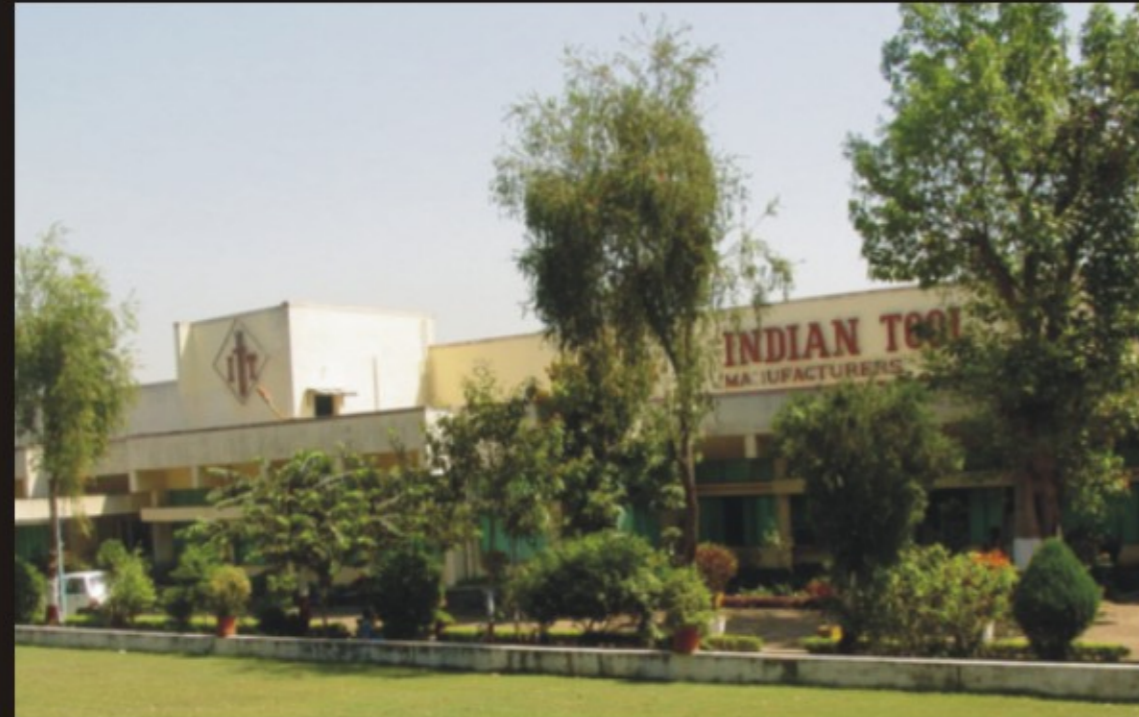
UNIT NO. 1 NASIK PLANT
